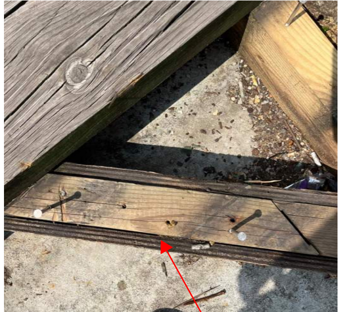
WOOD7 with plywood sisters for shimming 8/21/2024
