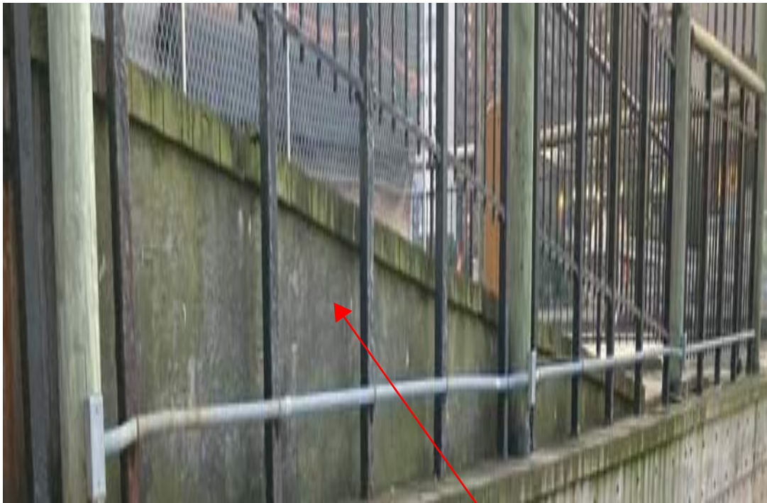
CONC10 Outside of North beam 8/21/2024
