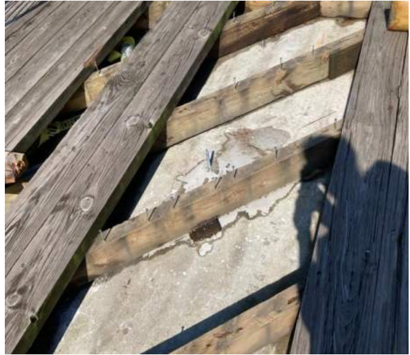
Typical sleeper framing 8/21/2024
