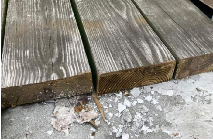
Decking is 2-1/2" of thickness and is pressure treated 8/21/2024
