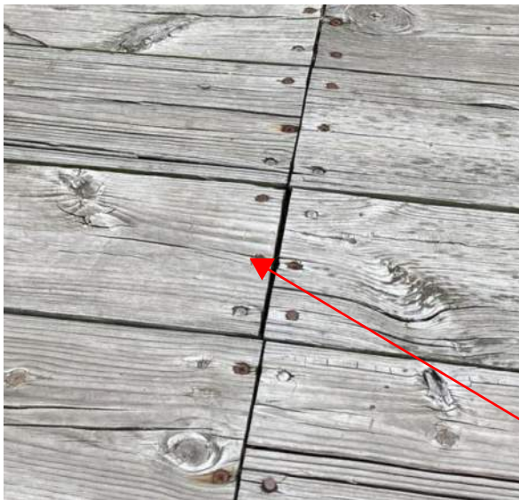
Most galvanized rusting hardware has been replaced with stainless steel ring shank nails
